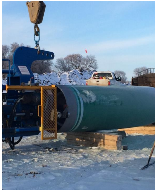
Counter bore on pipe 805 + 400
