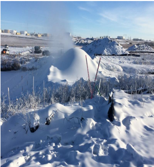
Making snow for ice bridge across Pipestone Creek MB 1010
