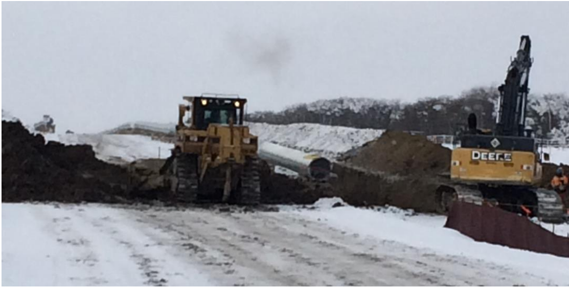
741 + 779 SF Excavating ditch
