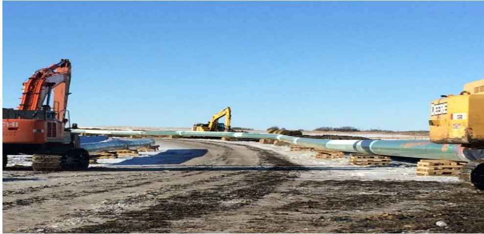
Product pipe ready for tie ins
